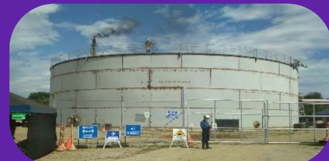
Sist. Contraincendios – Tanque TK2809
